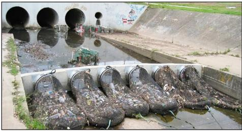
A series of nets used in a storm drain system in California to prevent trash from reaching local streams and the coast. Photo credit: Stormwater Systems, Inc.
